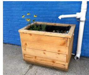
***Rainwater harvesting systems (cistern or rain barrel)***
