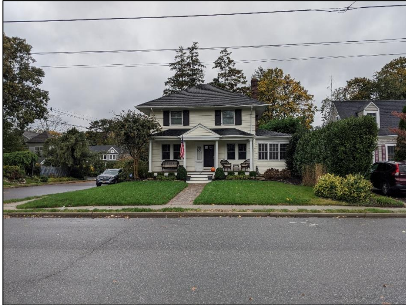
Front Elevation of 47 Lake Avenue
