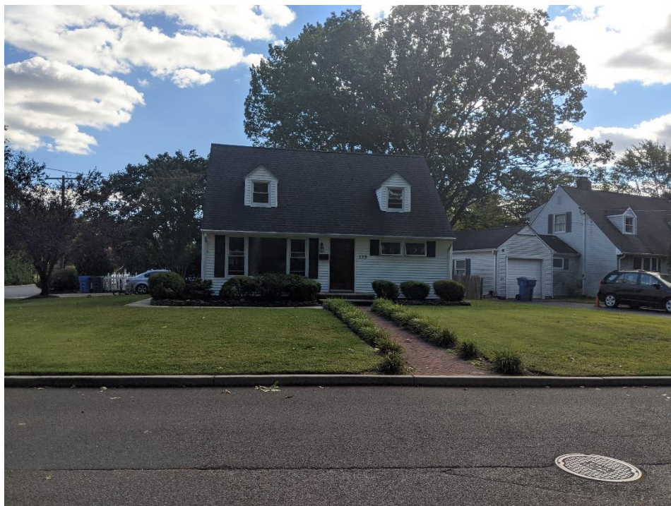
Photograph taken from Park Road
