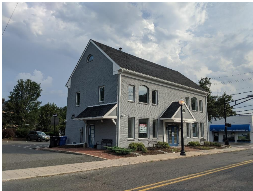
View of Front and East Side Elevation
