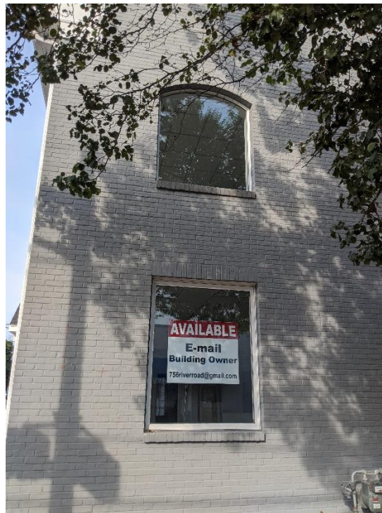
West Side of Building – Available Space Sign
