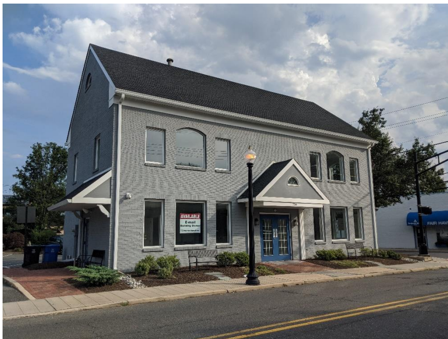
Front Elevation of Building Along River Road
