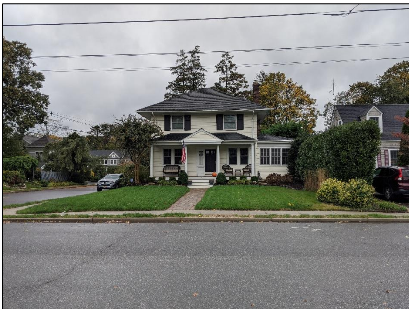
Front Elevation of 47 Lake Avenue
