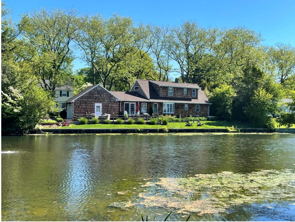
Rear of existing dwelling across McCarter Pond from Fair Haven Road
