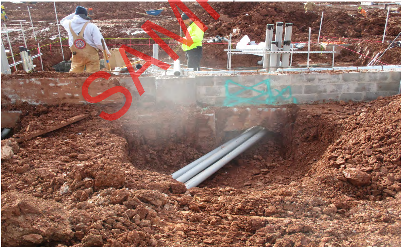
Secondary Conduit Run to Electrical Room
