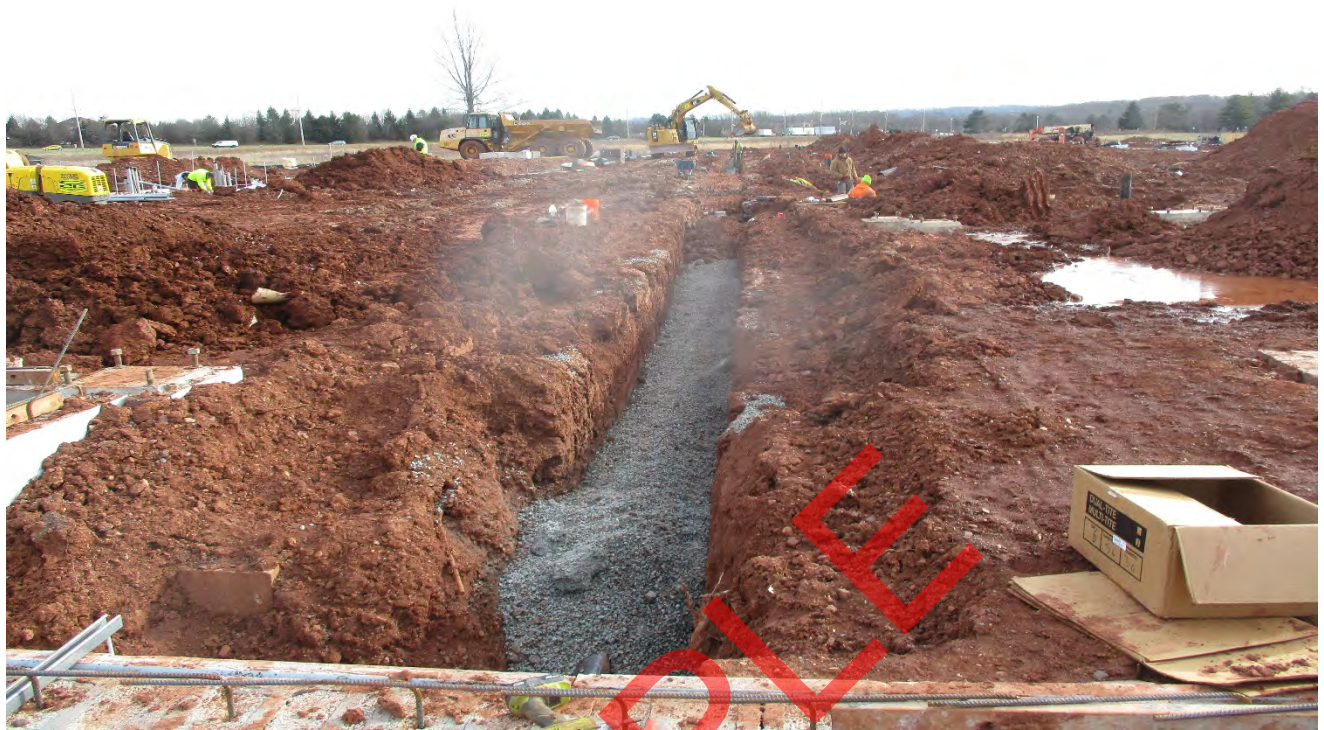
Under Slab Drainage Piping
